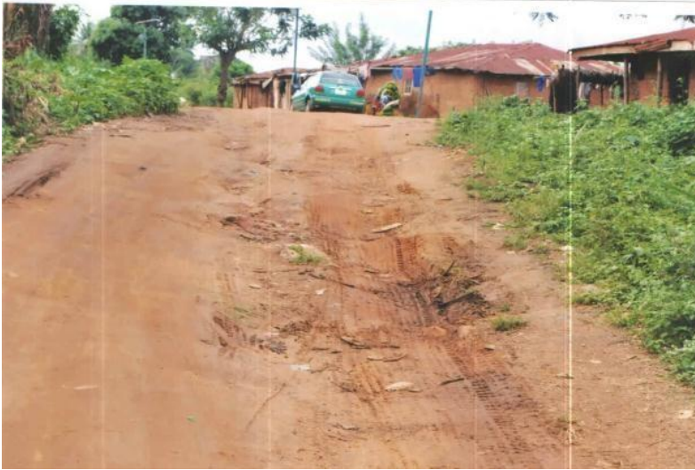
Plate 3: Earth Road from the main road linking AraromiIyin-Odo-Uro-Elemi
