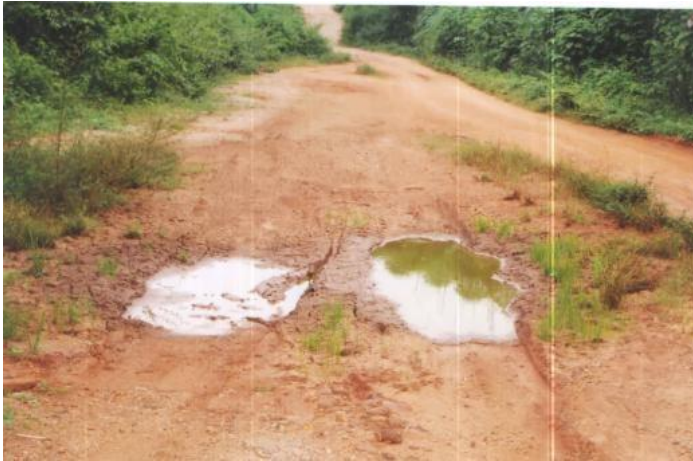
Plate 10: New Iyin road after FERMA office in Ado Ekiti. Source: Field survey, 2020
