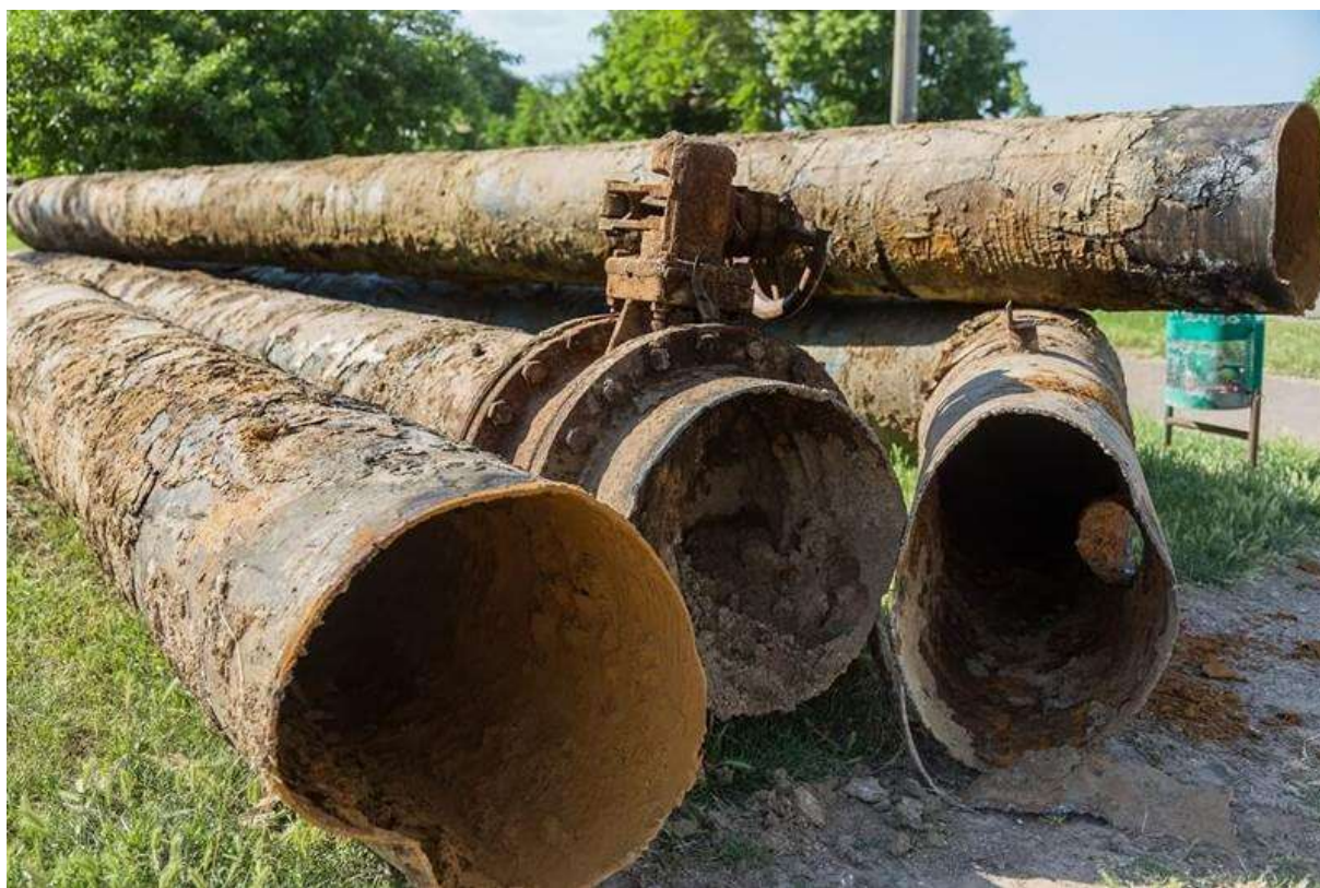
Figure 186: Picture showing corroded pipes (Corrosionpedia, 2023)
